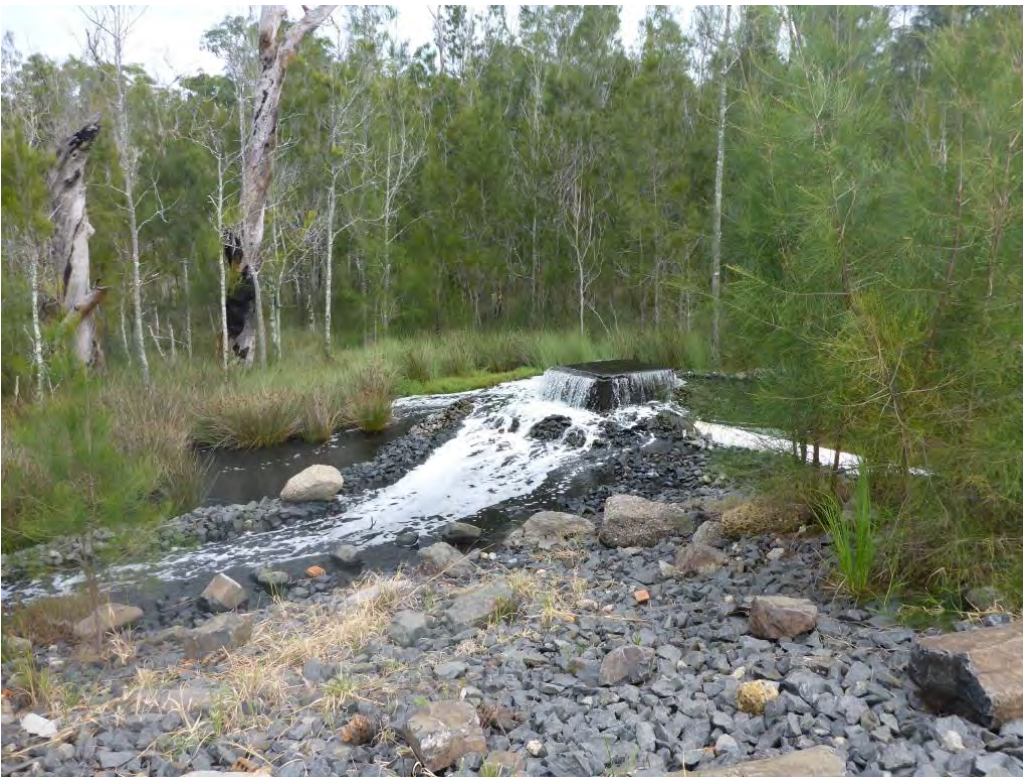
Photo 8 Licenced discharge point in operation
