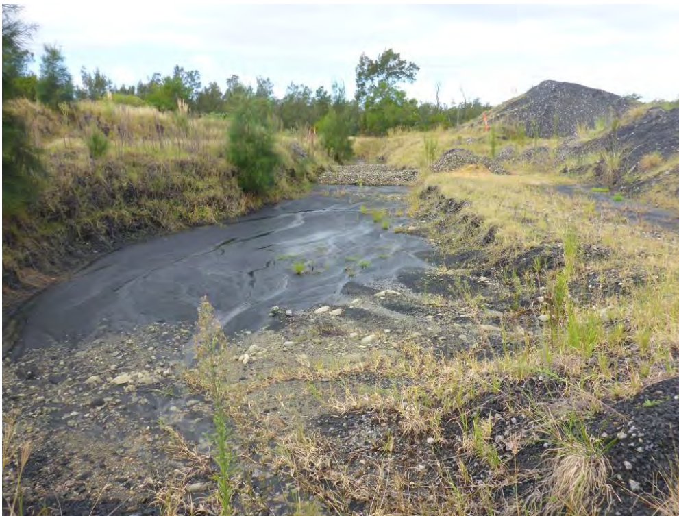
Photo 6 Coal Material in drain should be removed
