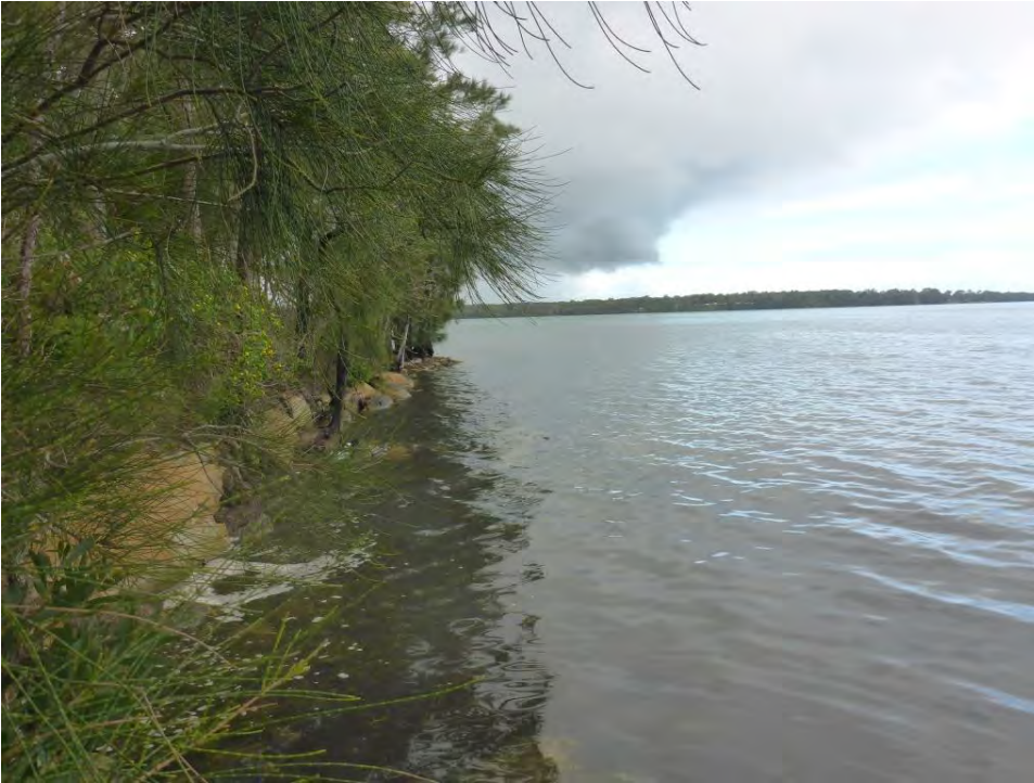
Photo 1 Previous Underground Mining Area – Lake Macquarie Shoreline
